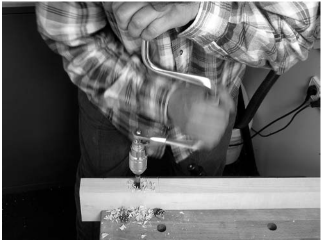
Pre-drilling the control cavity
